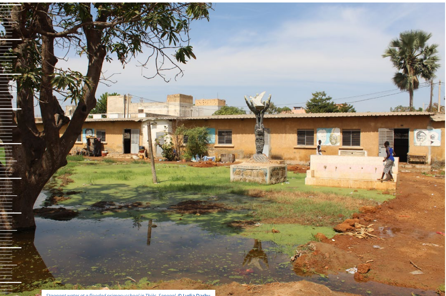
Stagnant water at a flooded primary school in Thiès, Senegal. © Lydia Darby
