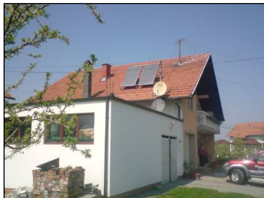
New solar systems installed on a home.
